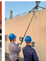
constructure inspection (WIFI real-time image transmission)
