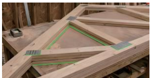
wood truss assembly
